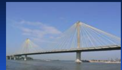
Clark Bridge at Alton - 060-0255
